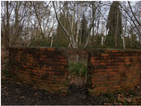
Photo 12. – Old brick structure (A7)
