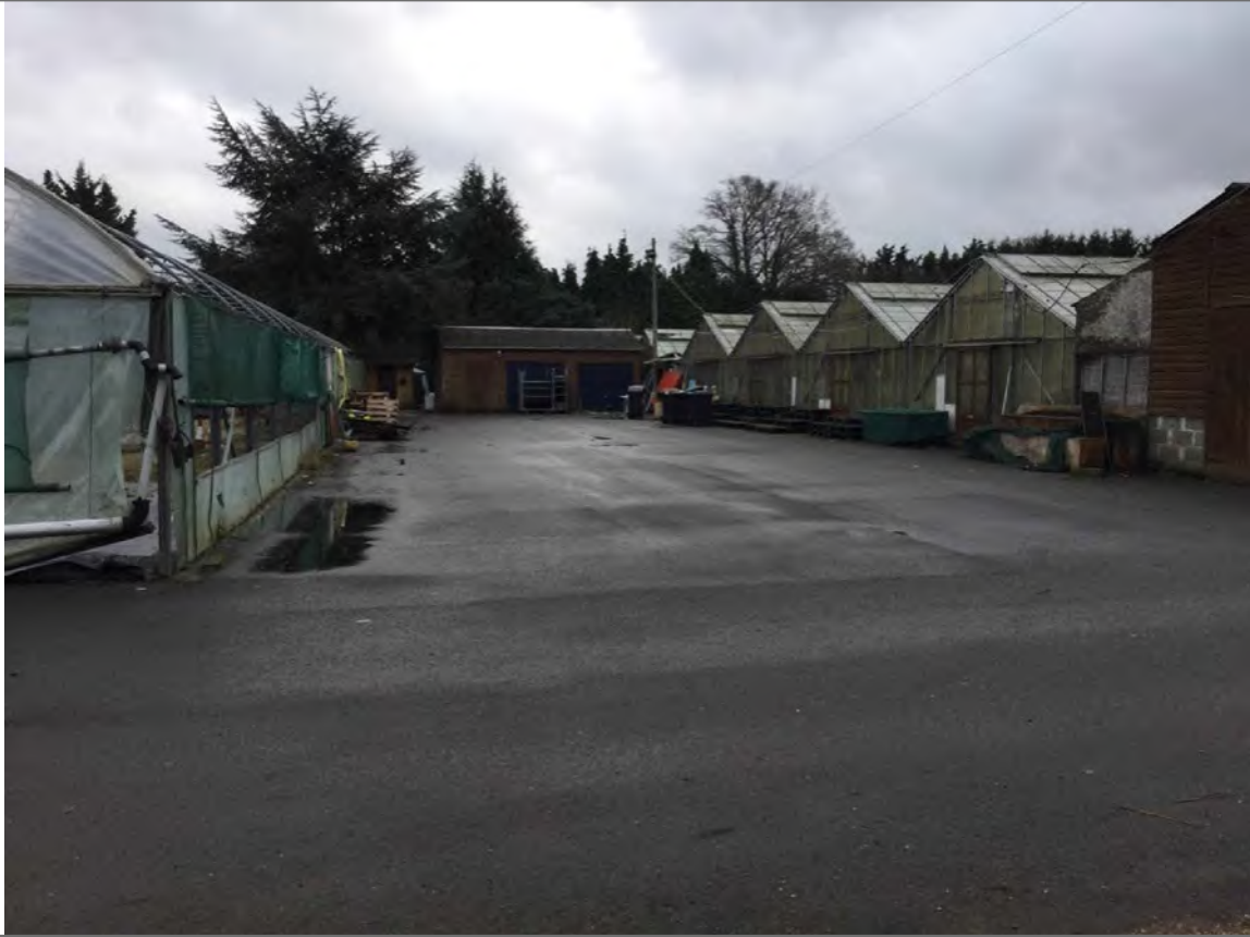
Photograph 1 Looking south into centre of the sub-area
