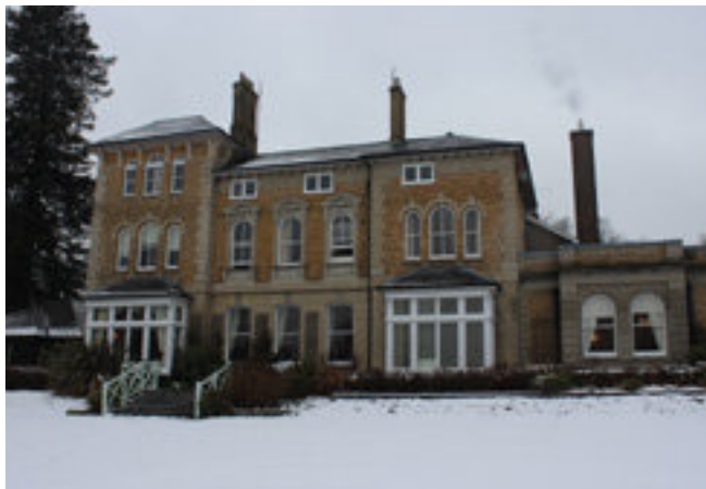
The Merlewood Care Centre in Virginia Water, like many buildings and structures on the Local List, has both historic and architectural interest
