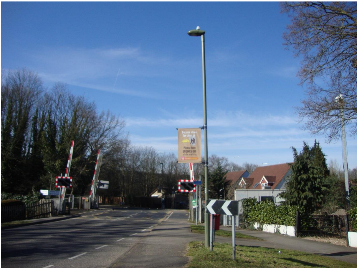
Figure 1 – Picture of signage erected at level crossing - Egham
