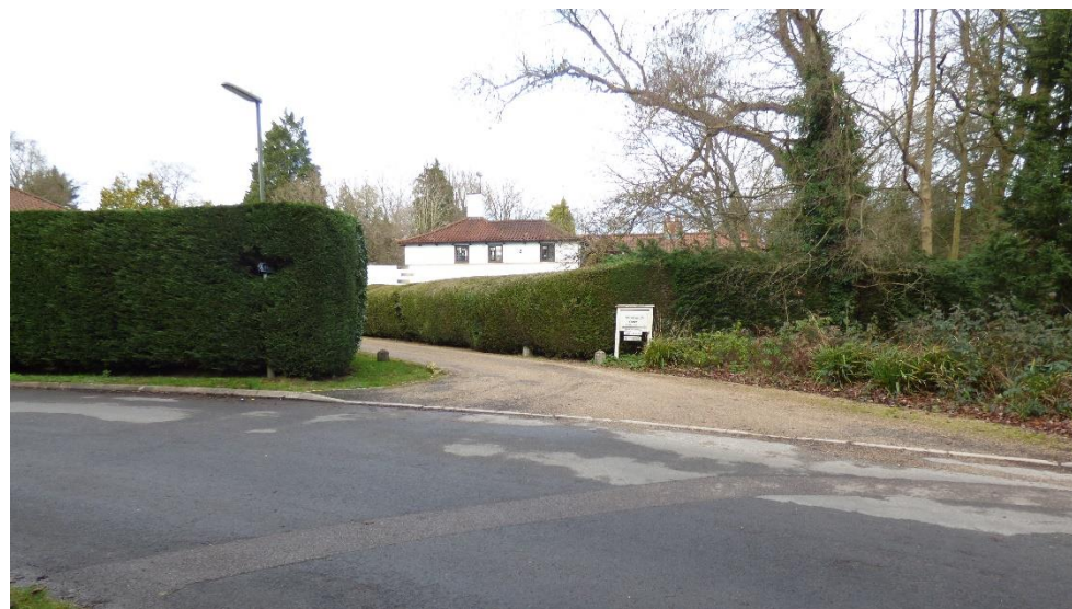
Figure 54: The listed lodge buildings on Ridgemean Road form the entrance to Ridgemean House.
