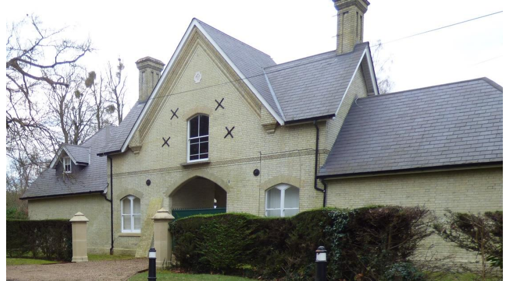
Figure 27: Castle Hill Stables features highly ornate brick and terracotta decoration on its gable and as part of its string course.
