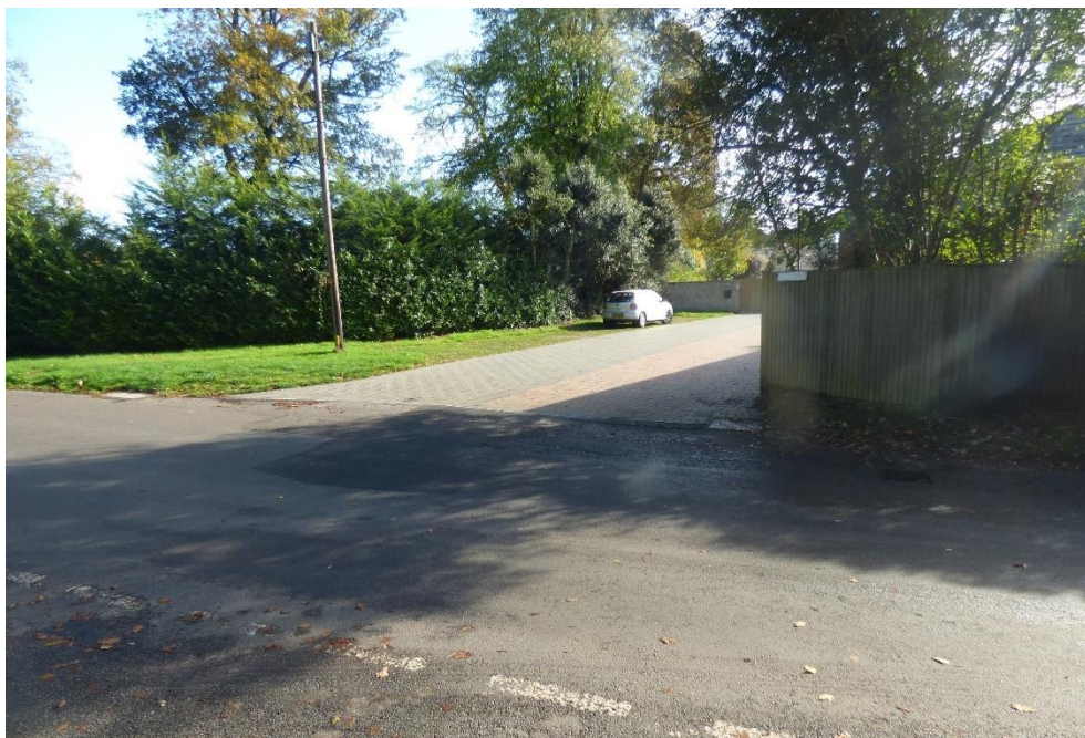
Figure 57: Double-width driveways and exposed close boarded fencing contribute to the urbanisation of the Conservation Area.
