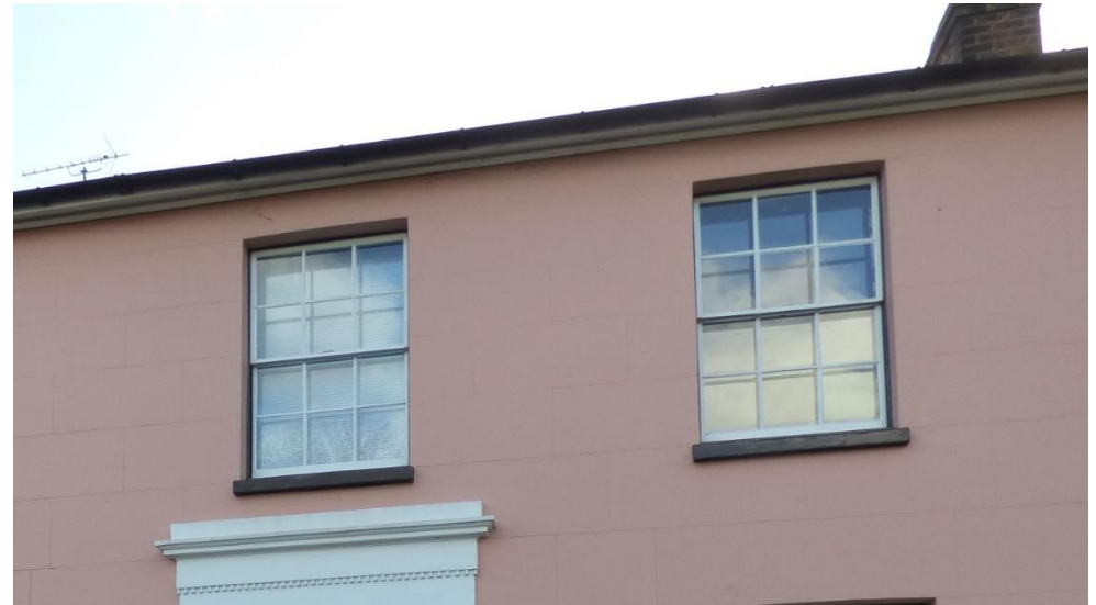
Figure 23: Examples of traditional six over six sash windows without horns in the Conservation Area.
