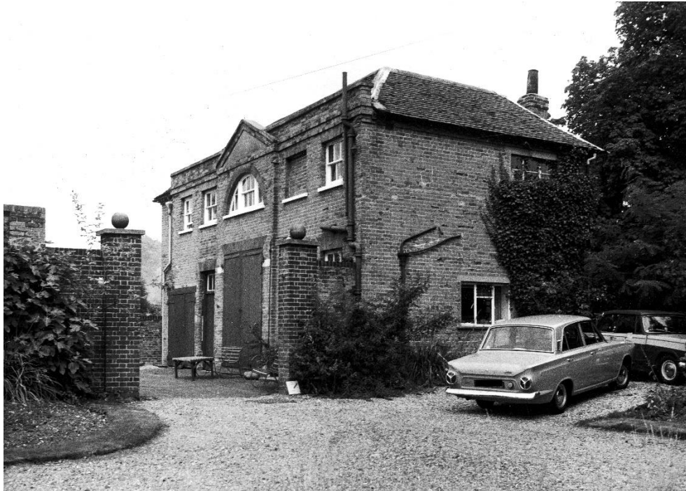
Figure 6: The Coach House to The Old House is a subservient building to the main house but is of a high architectural character. 8
