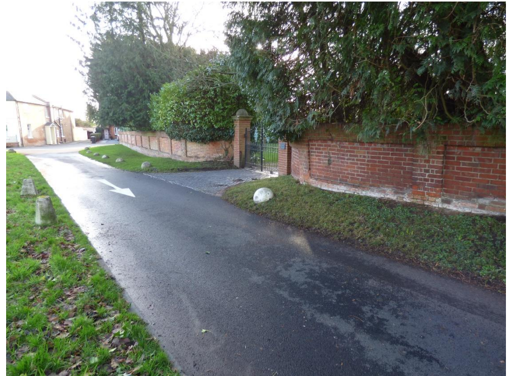
Figure 52: The brick wall to Crown House makes an important contribution to the Conservation Area.
