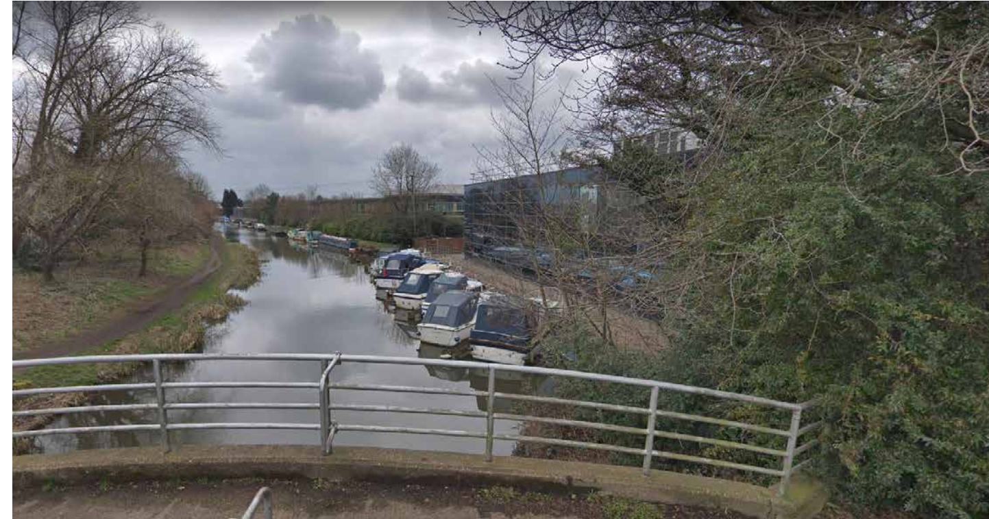
Existing View from Black Boy Bridge looking south
