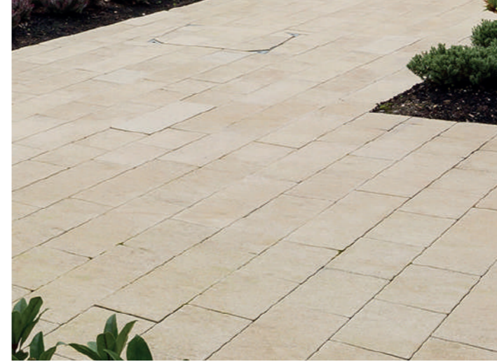
Concrete flag paving to access paths and outdoor social spaces
