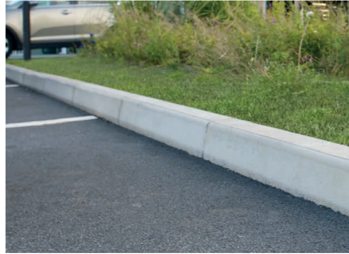
Raised and drop concrete kerbs
