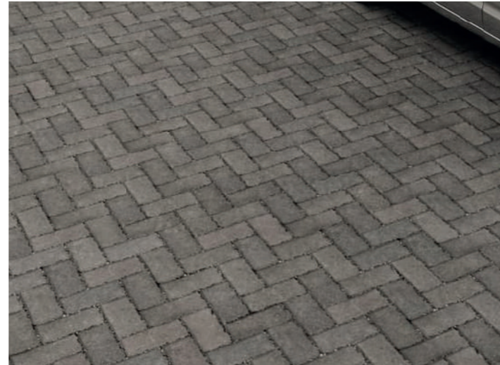
Permeable block paving to internal roads
