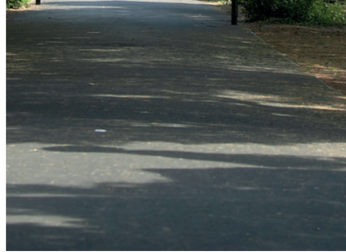
Asphalt footway surrounding site
