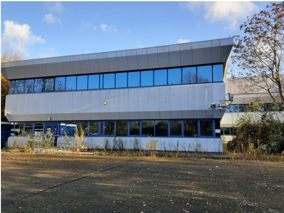
Photograph 4: Building B1 within the northern parcel
