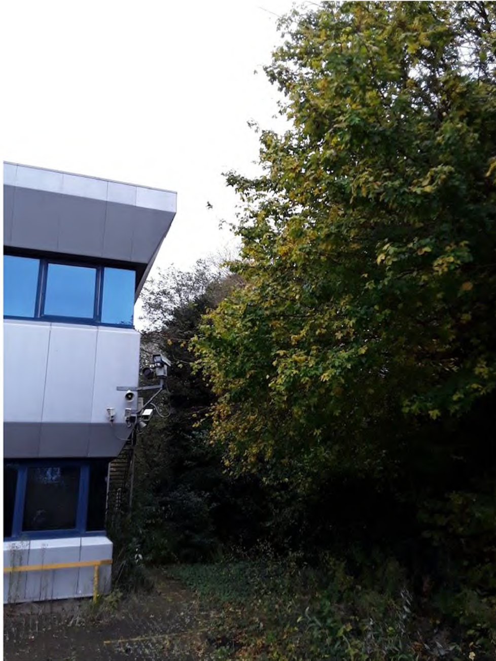
Figure 3 - Northern side of business park (looking North along G3)
