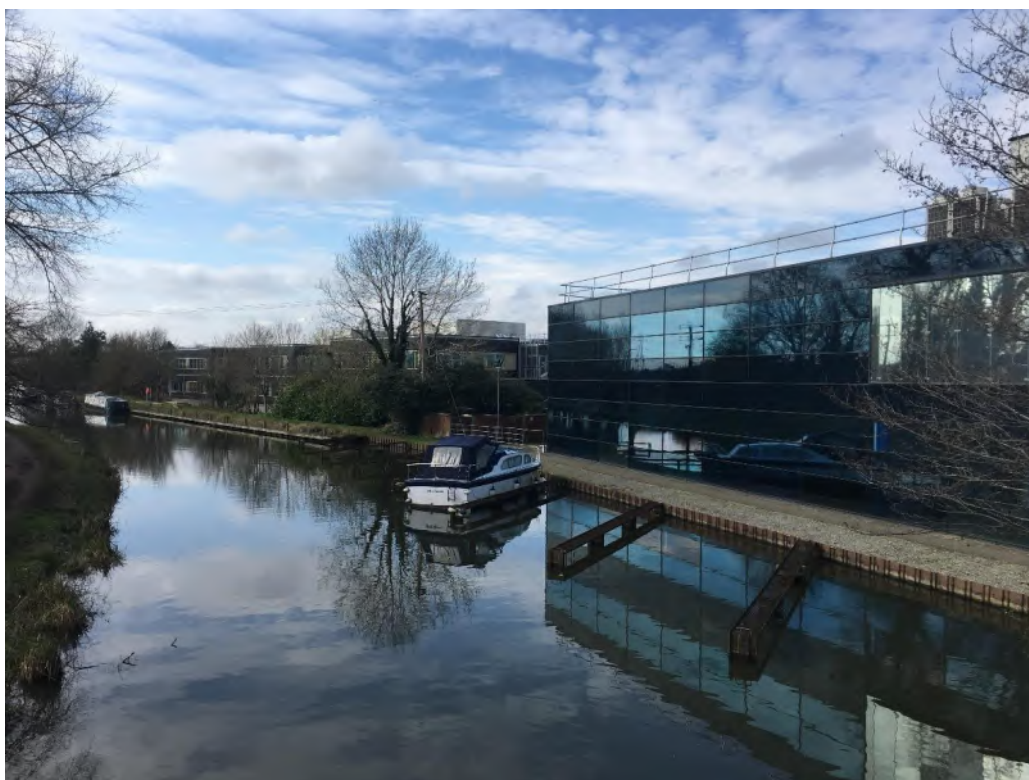
Figure 10: View towards the Site across the Wey Navigation Conservation Area, from the north-west, March 2022
