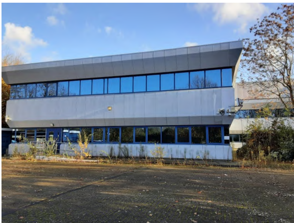
Photograph 4: Building B1 within the northern parcel
