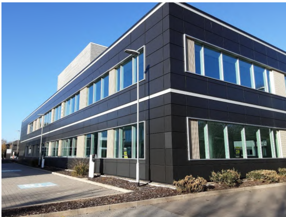
Photograph 3: Example of buildings in the southern parcel (building B6, Figure 1)
