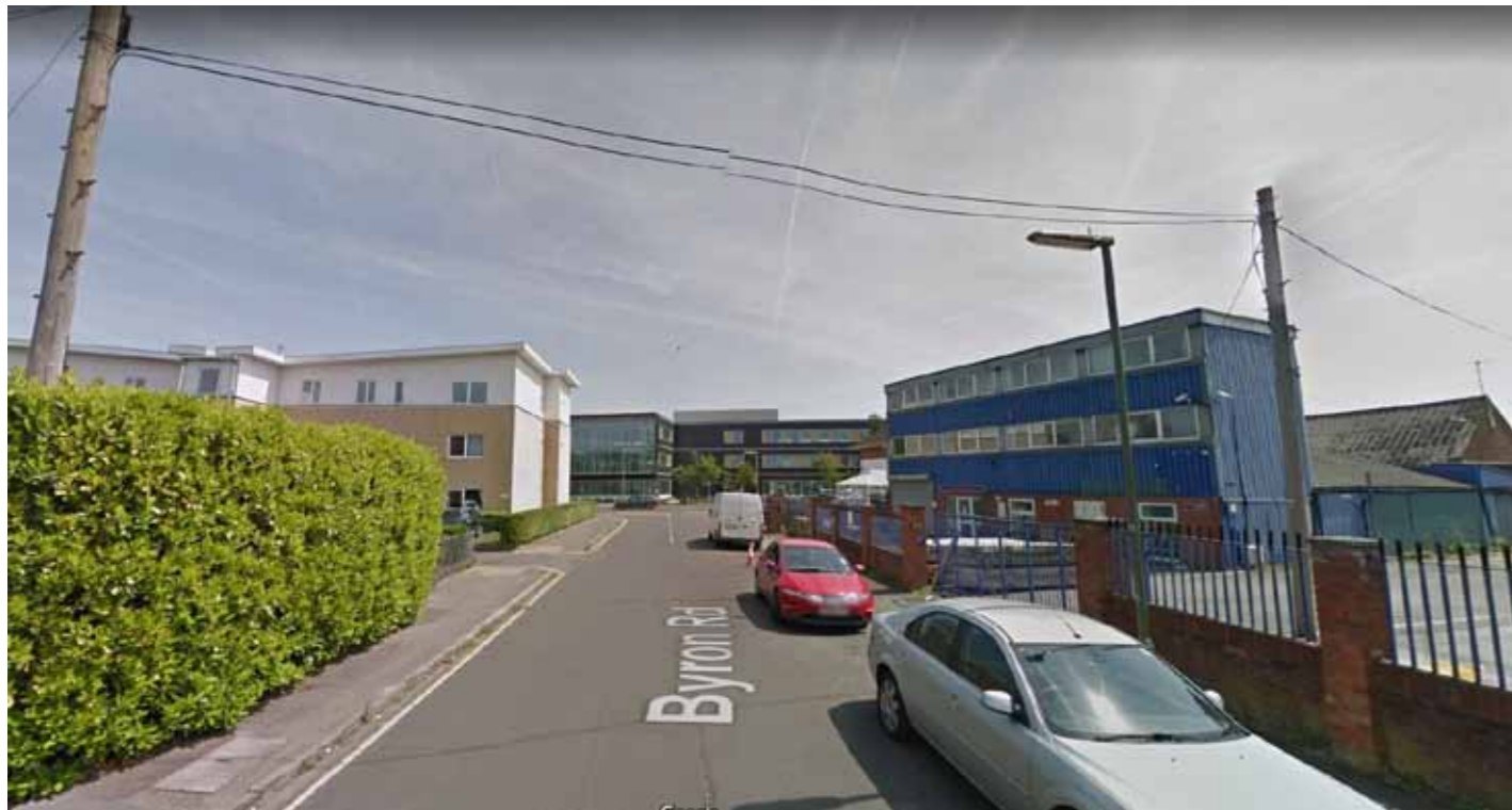
Existing View from Byron Road
