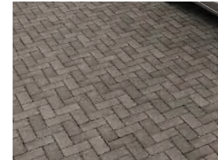
Permeable block paving to internal roads
