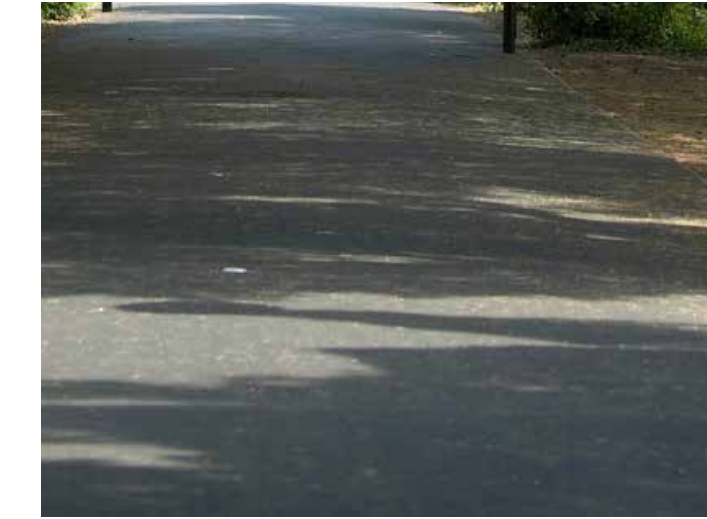
Asphalt footway surrounding site
