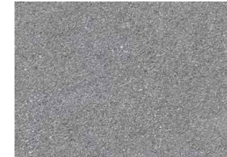
Asphalt parking bays
