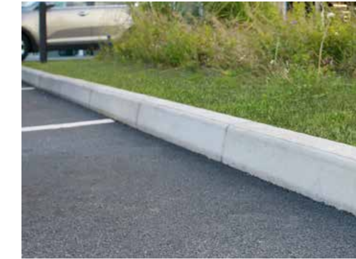
Raised and drop concrete kerbs
