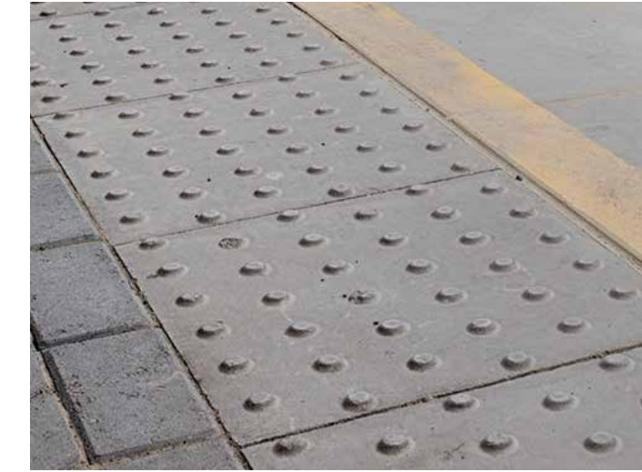
Tactile blister paving demarcating changes in level
