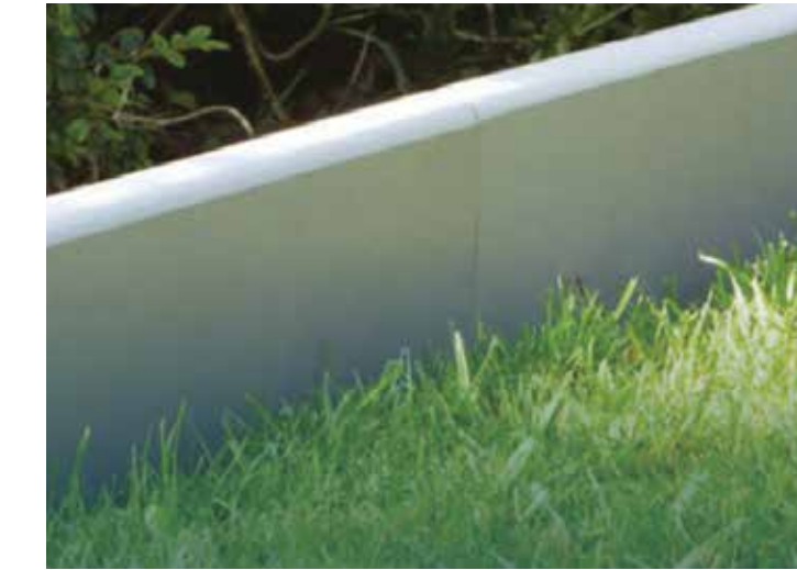
Concrete pin kerb edging
