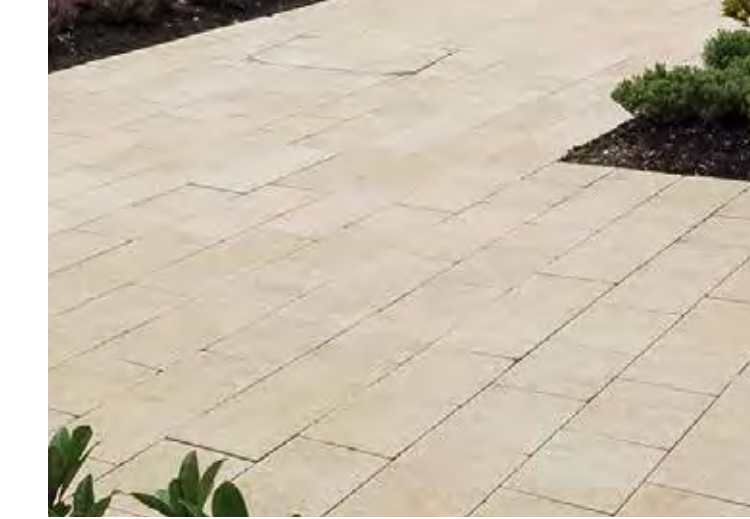
Concrete flag paving to access paths and outdoor social spaces
