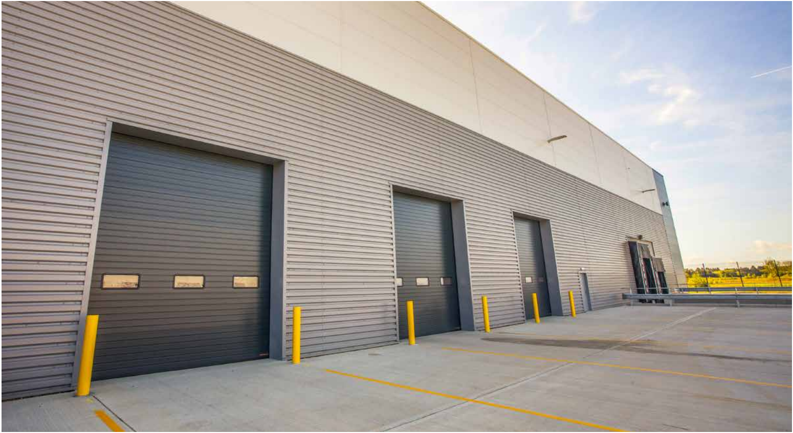
Structurally steel portals spaced at 8m provide maximum material efficiency in terms of steel sizing and structural tonnage. 8m grids also work most efficiently with industrial door coursing which is spaced at 4m.
