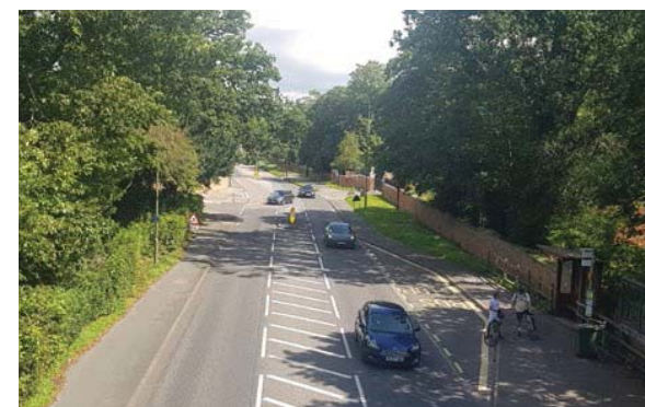
Figure 126. View of Egham Hill from footbridge
