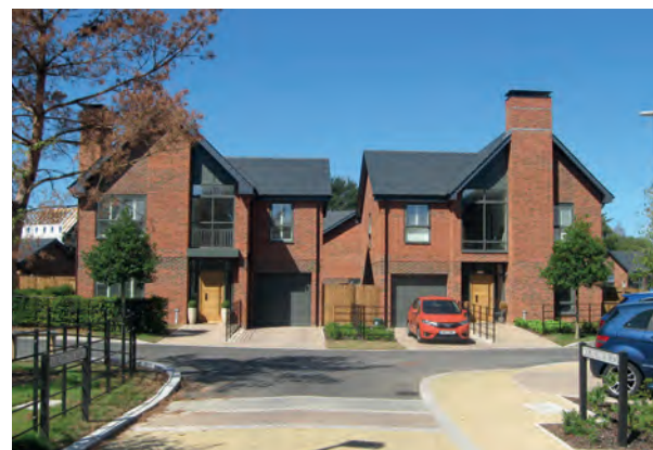
This intersection at Longcross North shows the transition from a tertiary street (with a variation of surface materials) into a secondary residential street (with tarmac carriageway), where houses are set back from the road by front gardens and parking in front of garages.
