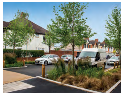
Rain garden swales with low maintenance planting are designed as part of this residential street in Grangetown, Cardiff.
