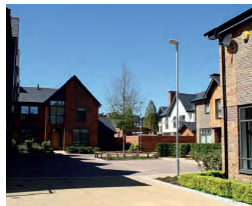
Development at Longcross successfully integrates small areas of parking within the street environment whilst maintaining access for residents and including elements of landscaping to help break parking areas up.
