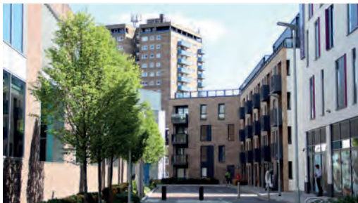
Addlestone One is a good attempt at contemporary residential development.
