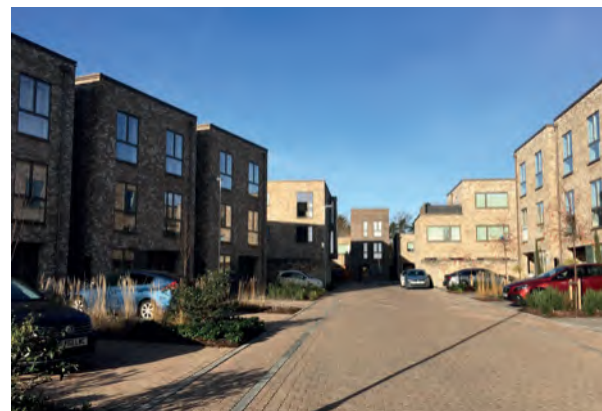
Clear and simple block structures lead to clear and simple street hierarchies, enabling residents and visitors to easily orientate themselves within a development. In Ninewells, Cambridge, a communal shared surface street is overlooked by the surrounding houses.
