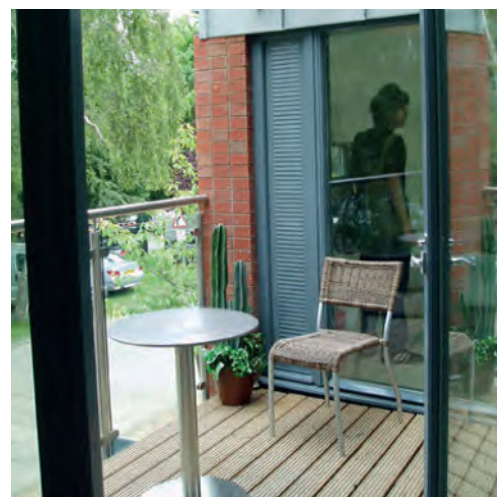
Inset balconies for flats and apartments give a better sense of privacy and are more likely to be used than protruding balconies.
