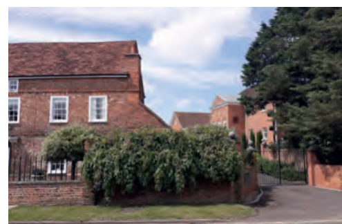
Renalds Herne/TASIS School, Thorpe-This Grade II listed building was purchased and renovated as part of the wider school development and now forms an important feature within the school site.
