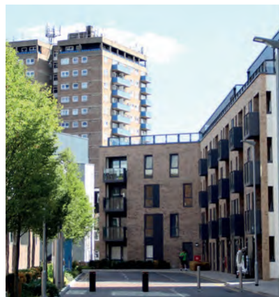
This four-storey apartment building in Addlestone provides enclosure and guides you round the corner, while its partially protruding balconies creates visual interest.
