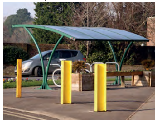
This cycle parking near Haywards Heath town centre is visible and sheltered. The run-off from the roof waters the planters around the cycle parking.
