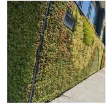
Green Wall Units: C, D & E
