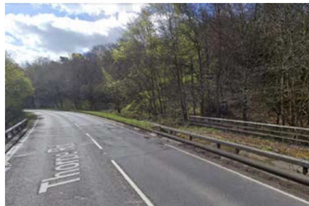
Figure 91. Thorpe By Pass on the M3 bridge and St Ann's Hill Woodland. Source: Google Street View
