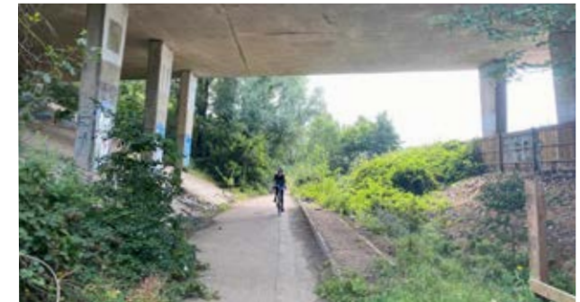
Figure 78. Route underpass allows for grade separation from Staines Road.
