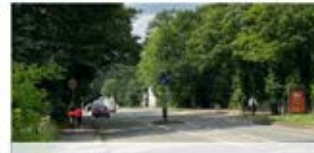
Figure 1.15 Virginia Water crossing (Sustrans)
