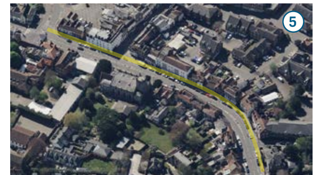
Figure 85. Two-way cycle track along southern side of the B375 (image credit: Bing Maps)
