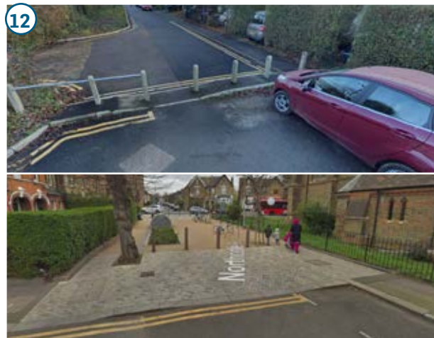
Top: Existing modal filter on Alexandra Road. The dropped kerb is narrow and the footways are restricted by on-street parking.
