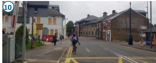
Chertsey Railway Station Poor pedestrian and cyclist provision on the approach to the railway station.
