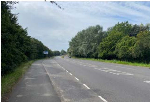
Figure 65. Staines Road with shared-use path at footway level.
