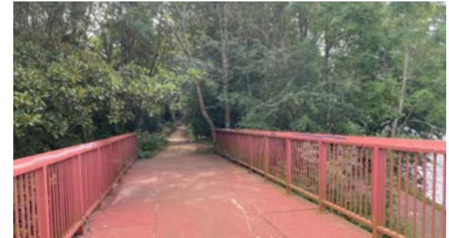
Figure 77. Existing route facilities at Monk's Walk.
