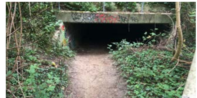
Figure 79. Partly-buried route underpass below the M3 linking Monk's Walk to Chertsey.
