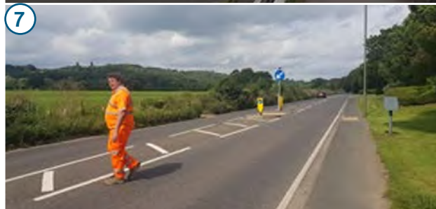
Top: Existing uncontrolled crossing on Egham By-Pass. Bottom: Existing uncontrolled crossing with a refuge island on Windsor Road
