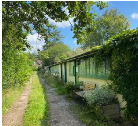
Dell Park Stables and Courtyard Workshops
