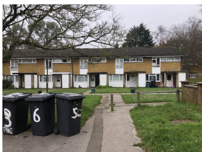
Front Doors Accessed by Path
