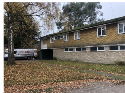
Property with Boarded Windows
