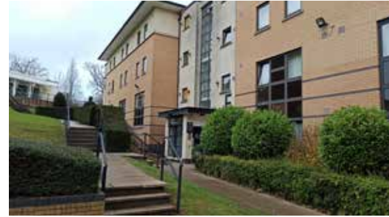
Figure 69: Change in level on site
