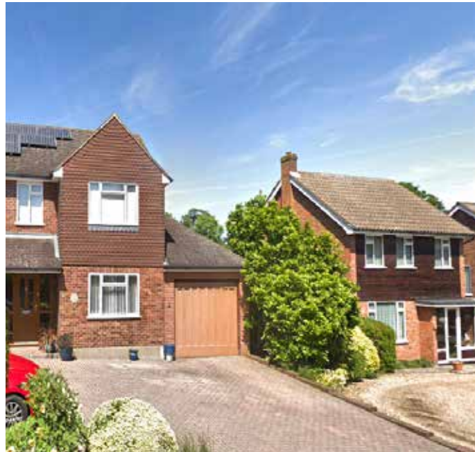
Figure 31: Alderside Walk. On-plot parking on garage
