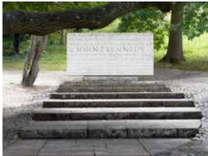
Figure 24: John F Kennedy Memorial, Listed Grade II
