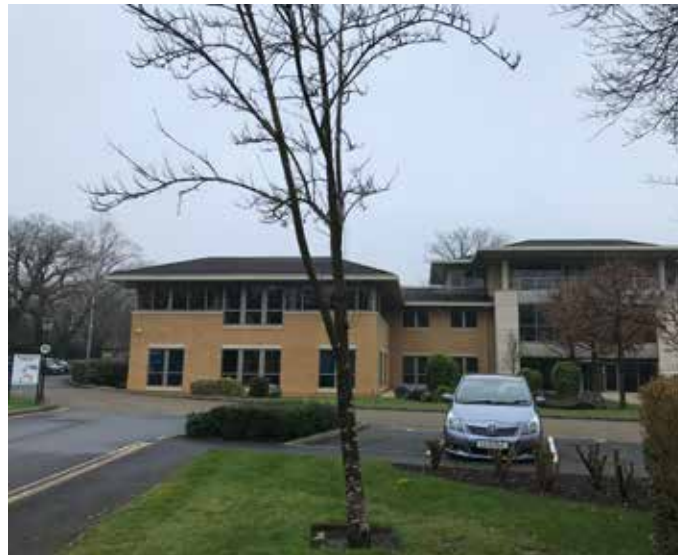
Figure 39: Blay's House viewed from the car park to the south
