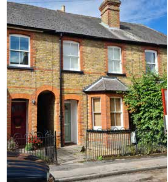
Figure 07: Victorian property with feature bay windows, Harvest Road
