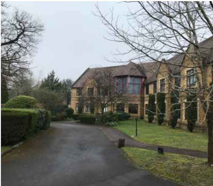
Figure 45: Trees play an important role in enclosing and screening the built development on site.
