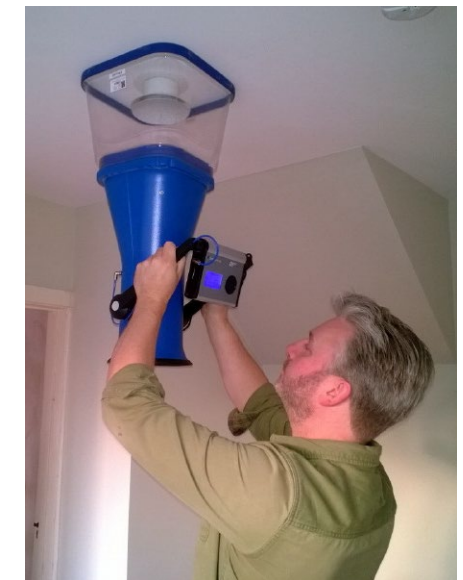
Flow rate measurement: image of MVHR system being commissioned (Source: Fourwalls)
