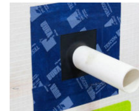
Airtightness grommets need to be used so that service penetrations do not increase air permeability (Source: Pro Klima)
