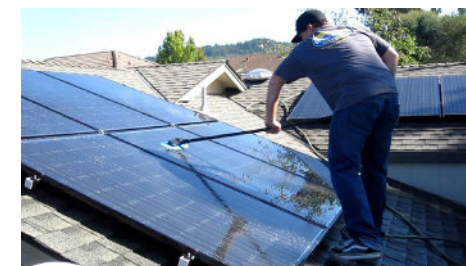
PV panels need to be cleaned at least once per year. (Sources: EasyAcc, Amethyst Cleaning)
