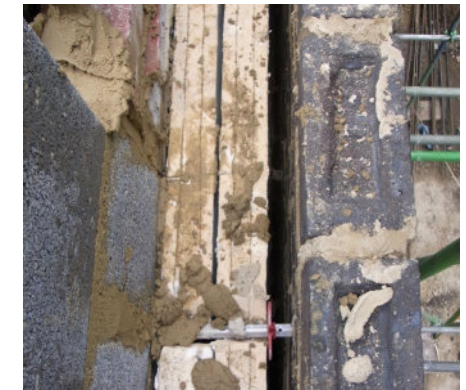
Left: an example of good Expanded Polystyrene insulation installation. Right: An example of poorly installed partial cavity installation, loosely fitting, and cement dropped atop and inside cavity (Source: Etude)
