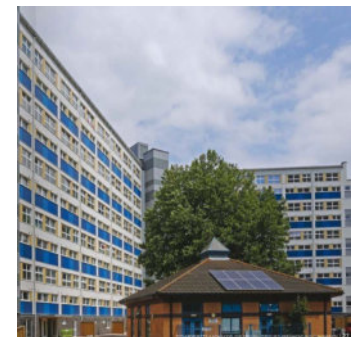
Wilmcote House, Plymouth (Source: ECD Architects)
