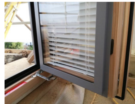
Replacement triple glazed windows (Source: Internorm)
