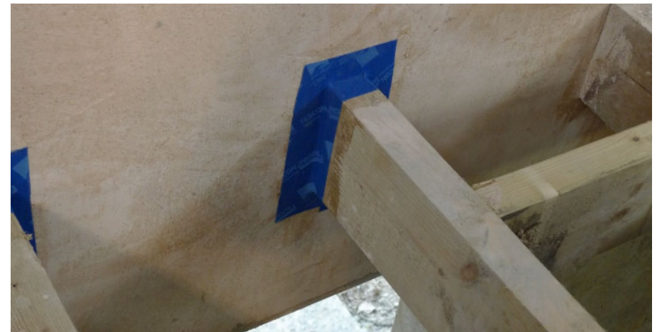
Applying airtightness tape to joist ends is a common measure required to achieve good airtightness in existing buildings. Large gaps may need filling with mortar first, and remember to apply a suitable primer. (Source: Ecomerchant)
