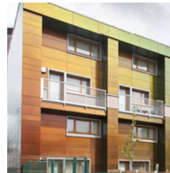
Ernley Close, Manchester (Source: 2e Architects)
