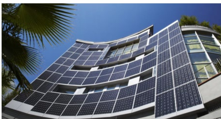
South facing solar facades produce around 15% less energy than an East/West concertina array, but generate more electricity than an East/West array in winter months. For buildings with heat pumps, this can be a great match. (Source: Solarbuildingtech.com)
