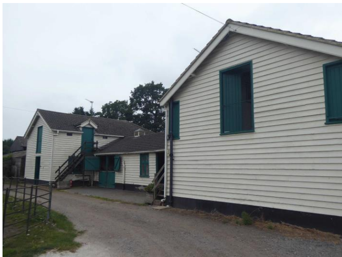
The stables looking west.
