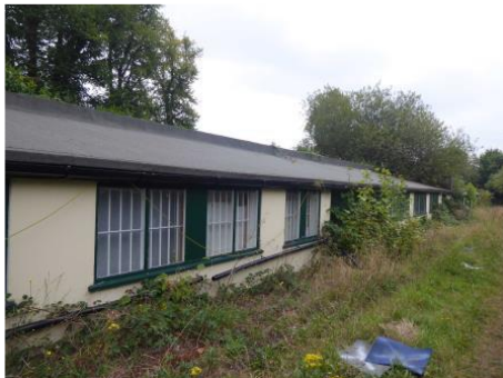
Top the north entrance to the walled garden (exterior). Middle, the interior of the garden wall with greenhouse brackets. Bottom the east range buildings.
