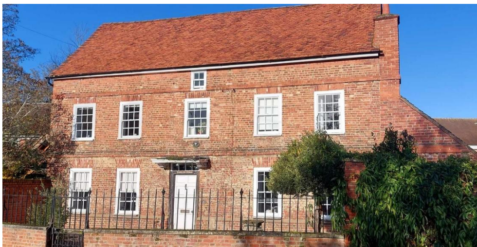
Figure 6: Renalds Herne, Coldharbour Lane shows a number of features that are typical of buildings in the Conservation Area including string coursing, sash windows with brick detailing above, the use of deep red brick and a panelled door with a case surrounding it and a canopy above.
