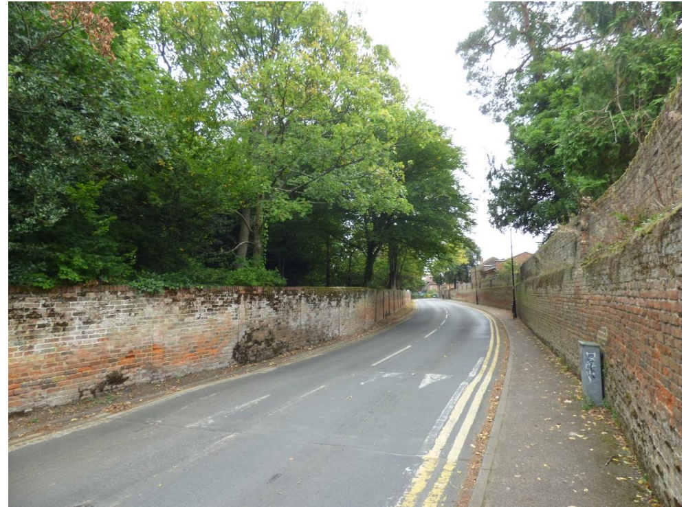
Figure 41: View 4 looking east along Coldharbour Lane.
