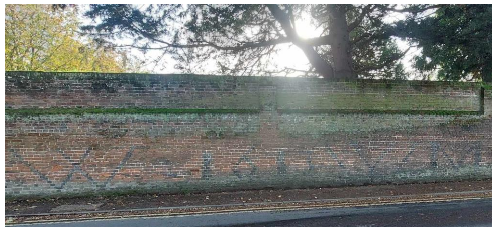
Figure 7: Diaper brickwork in the boundary wall on the south of Coldharbour Lane, spelling W 1613 W M.
