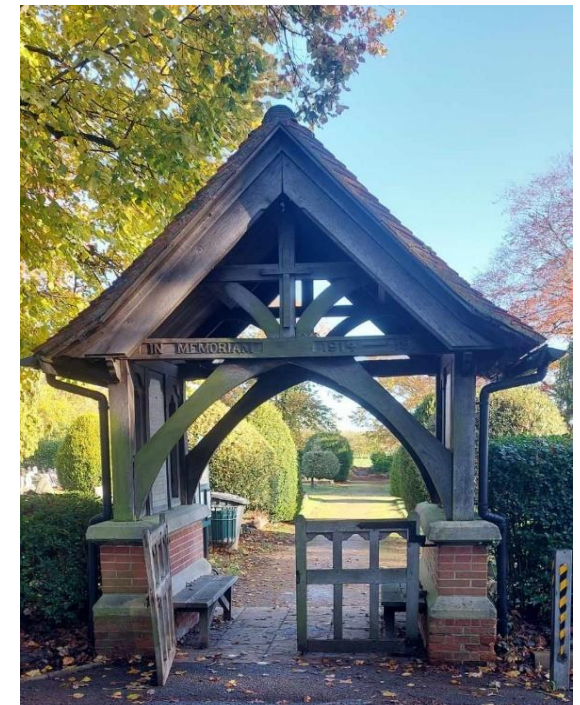
Figure 50: The locally listed Lych Gate at Thorpe Cemetery.
