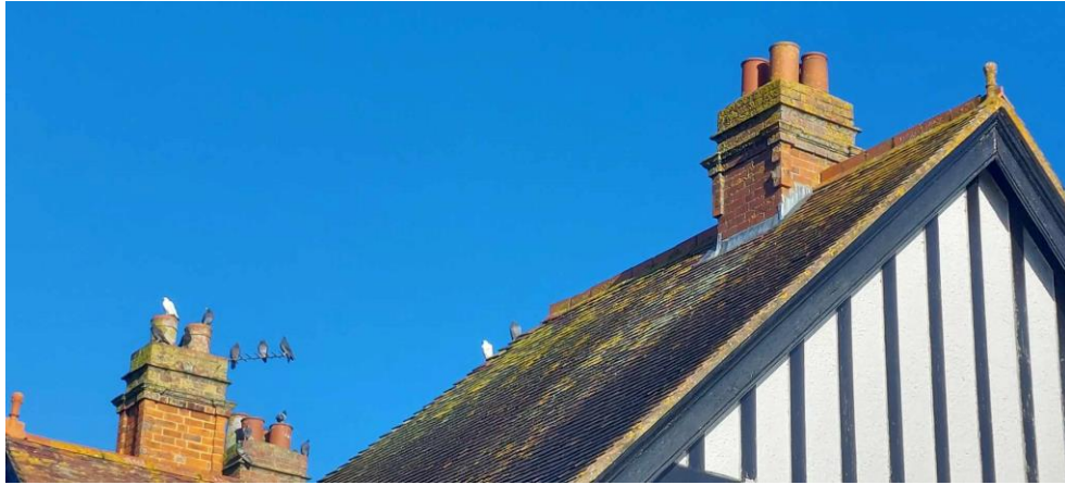
Figure 32: An example of a steeply pitched gable and brick chimneys.
