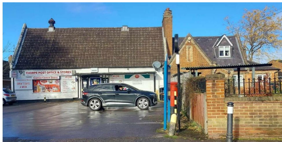
Figure 66: Thorpe Post Office, which has been insensitively changed over time.
