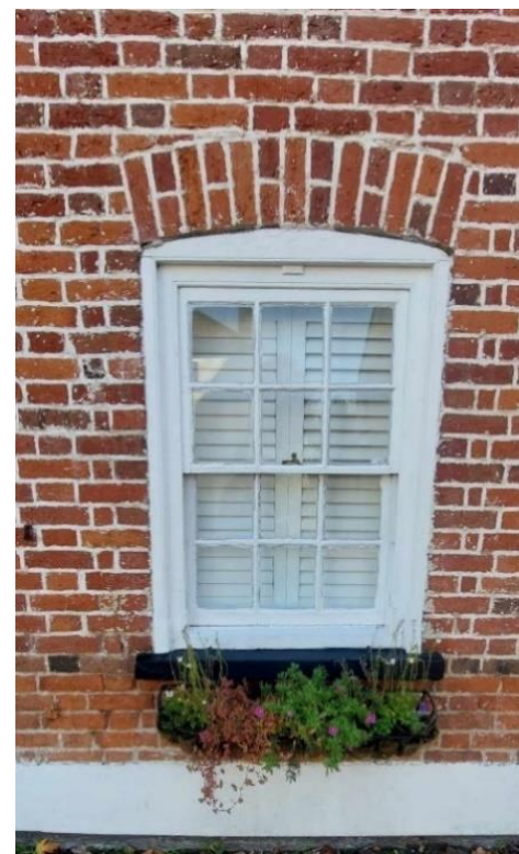
Figure 28: A square headed, timber-framed sash window with brick detailing above.
