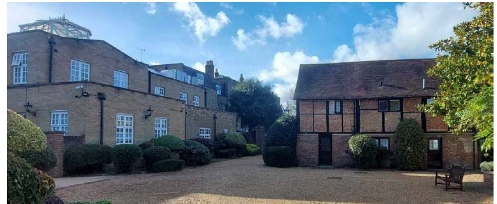
Figure 25: An example of yellow brick used on some of the TESIS school buildings, as well as an example of a timber framed building in the Conservation Area.
