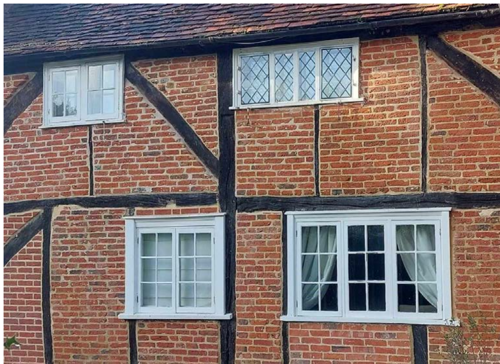
Figure 29: Timber-framed casement windows.
