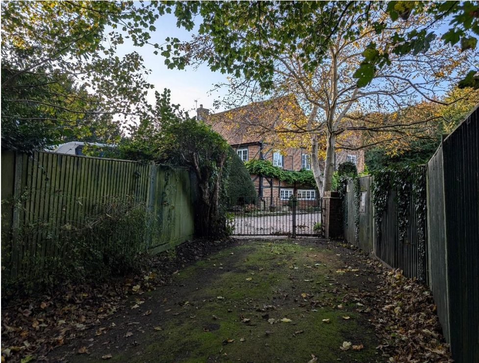
Figure 55: An example of a large residential property on Norlands Lane, set back from the road on a generous plot.
