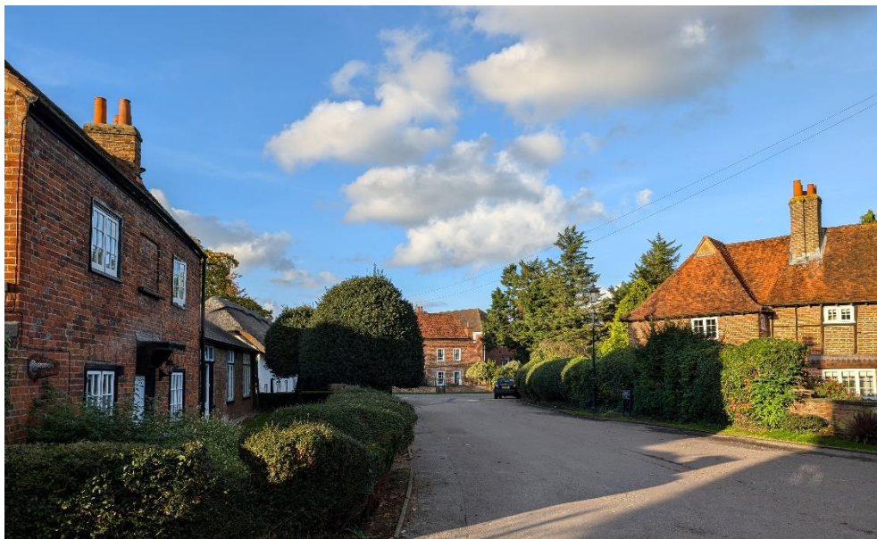
Figure 59: Some of the buildings along Church Approach, with Renalds Herne viewed in the distance.
