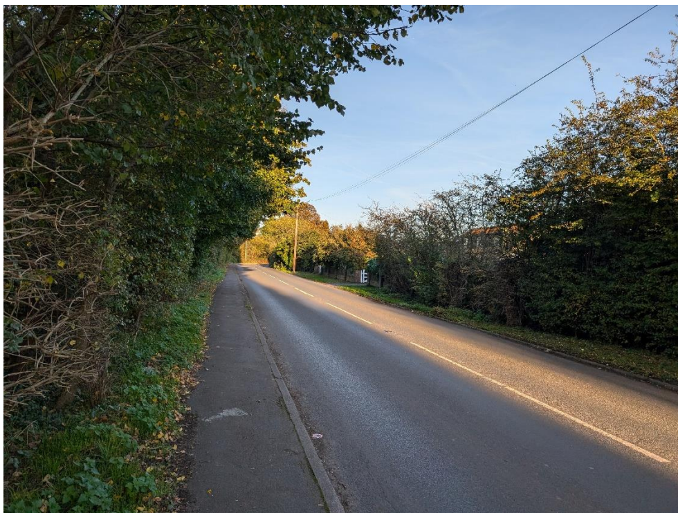
Figure 46: View 9 looking east along Coldharbour Lane from Thorpe Park Farm.
