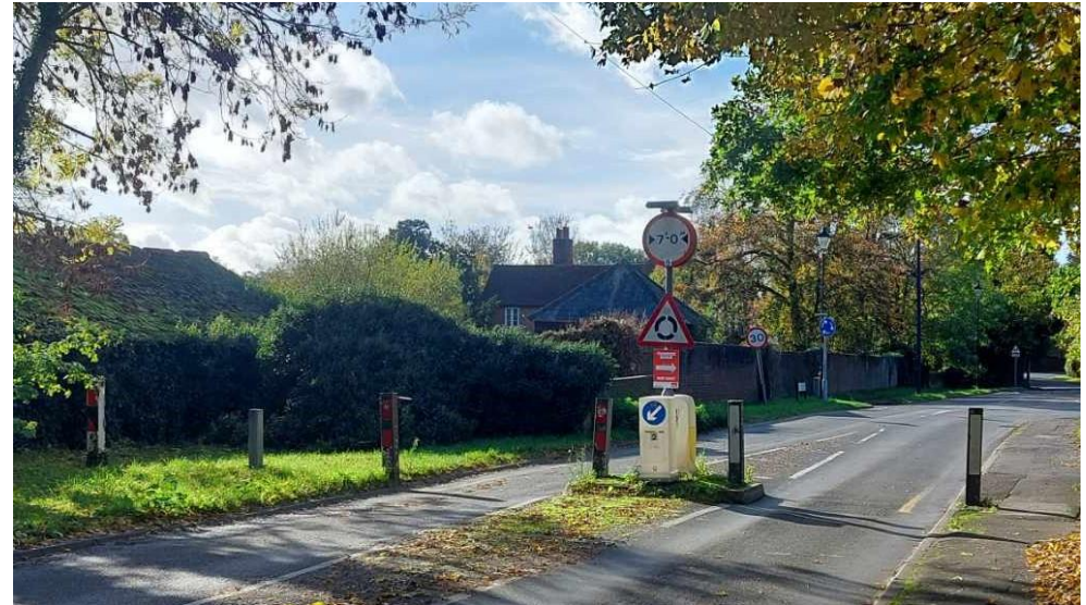
Figure 64: The series of posts and signs, which form a key 'gateway' into the village, detract from the appearance of the Conservation Area.
