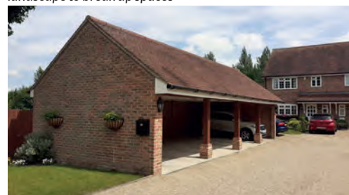
Blackhouse Farm, Thorpe: Provides a high quality, purpose built solution to help screen and break up parking areas within the wider development
