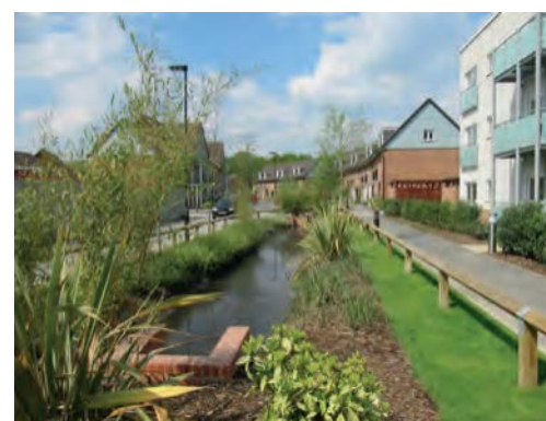
SuDS features in Watercolour, Surrey, are planted to provide biodiversity value and create an attractive environment.
