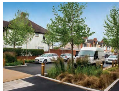
Rain garden swales with low maintenance planting are designed as part of this residential street in Grangetown, Cardiff.
