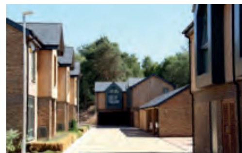
Positive example of a design matching meter boxes, integrating satellite dishes at eaves line, no unnecessary things on front elevations, and high quality doors to services/bin stores (Longcross)
