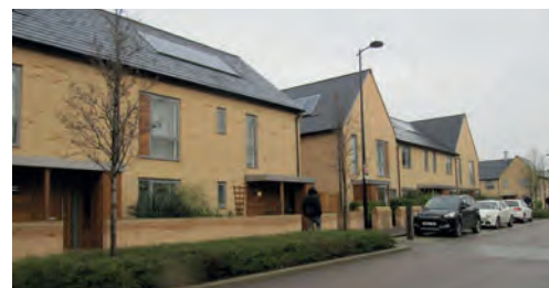
Parallel street parking incorporating material changes and landscape to break up spaces
