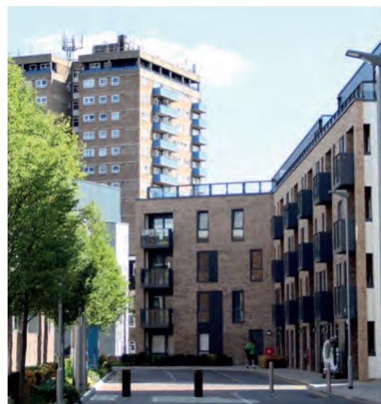
This four-storey apartment building in Addlestone provides enclosure and guides you round the corner, while its partially protruding balconies creates visual interest.
