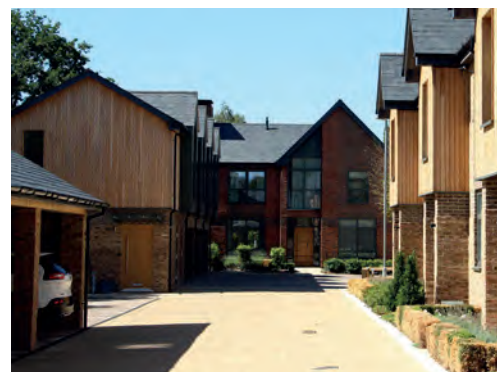
Development at Longcross shows care in the grouping of buildings, and in the coherence of individual buildings as they relate to one another and the space around them. Three dimensional detailing is integral to the design approach.
