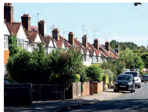
Regular projecting gable and chimneys with consistent materials in a residential street in Stroud creates a distinctive roofscape.
