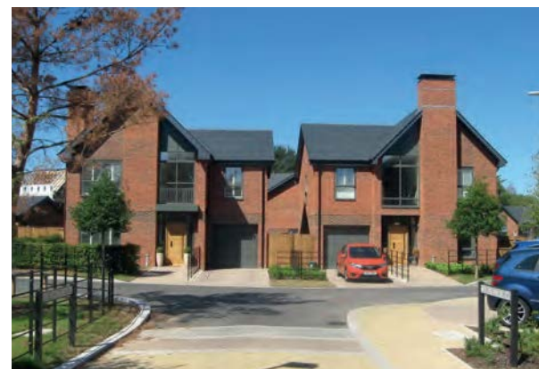
This intersection at Longcross North shows the transition from a tertiary street (with a variation of surface materials) into a secondary residential street (with tarmac carriageway), where houses are set back from the road by front gardens and parking in front of garages.
