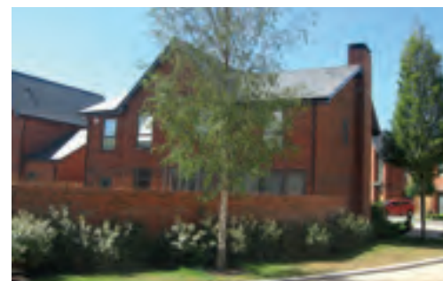
Positive use of consistent materials for boundary walls that complements the building.
