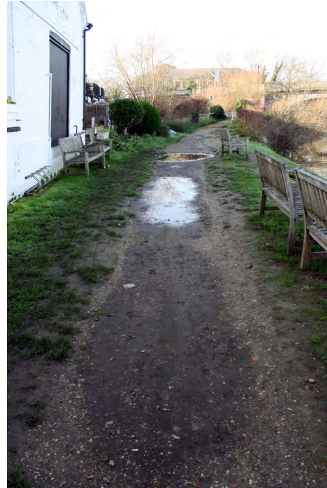
Muddy and puddled part of the Thames Path, which is suffering from erosion
