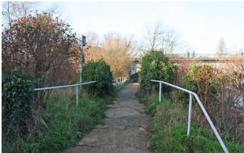
View looking west showing the footbridge at the western end of the Thames Path passing under Staines Bridge
