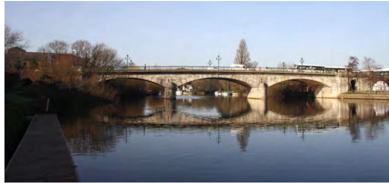
View of Staines Bridge from the Thames Path
