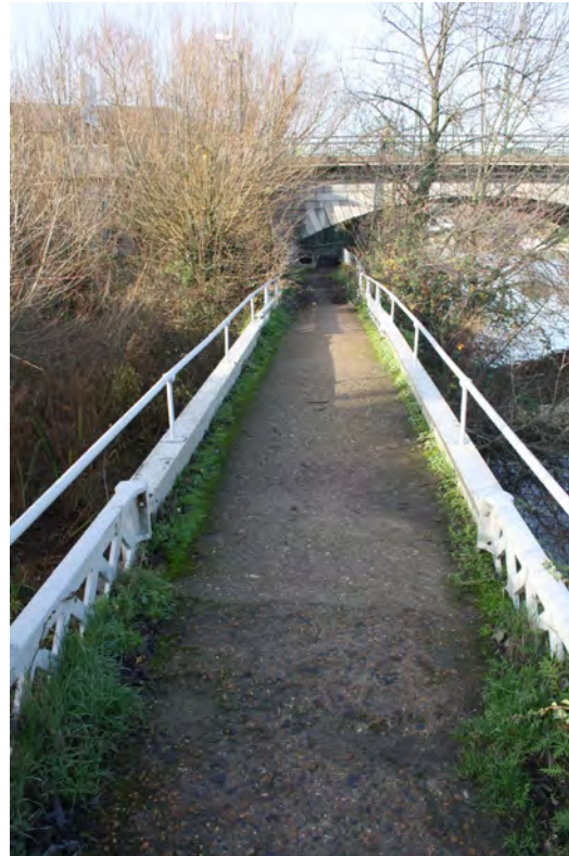
Low railings to Thames Path footbridge over an inlet
