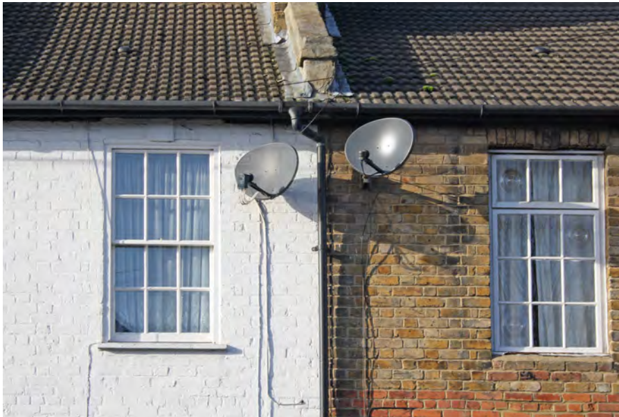
Examples of satellite dishes mounted to front elevations in Farmer's Road and the associated visible cabling
