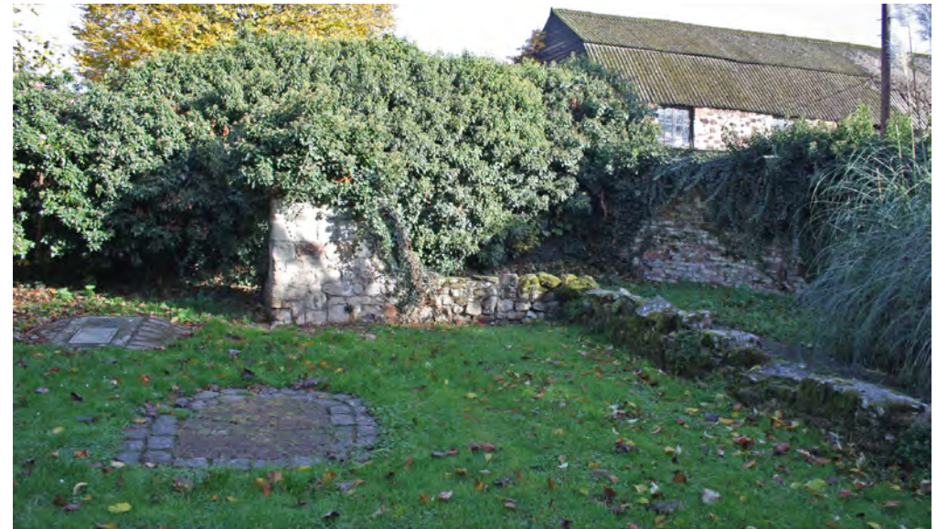
Former Abbey walls in the treed area to east of playing fields
