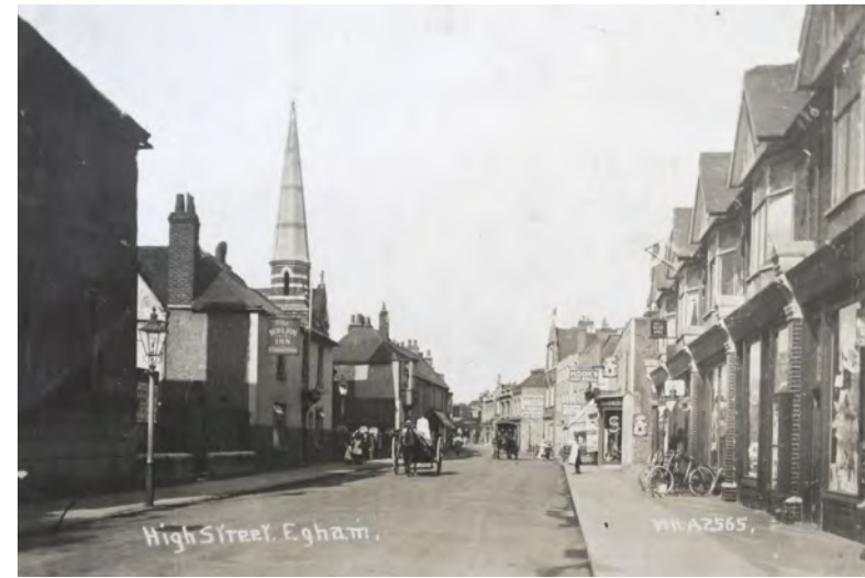
View of the High Street looking east showing the Literary Institute and the Red Lion on the left, undated [c.1910] (Egham Museum Trust, P 109a)
