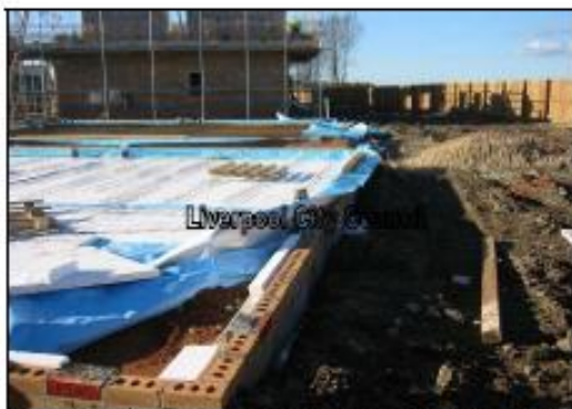
Use of non gas resistant DPM (blue backing colour) of same colour as gas resistant DPM (silver backing colour), with only gas resistant membrane used across cavity (to appear like gas resistant membranes after casting of slab. Sacrificial membrane absent with sand blinding filling granular void.
